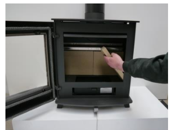
4. Remove the right hand side brick followed by the 2 rear bricks
