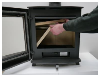
3. Ease the left hand side brick away whilst supporting the front baffle section with your other hand. Carefully manoeuvre both baffle brick sections out of the stove
