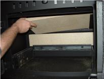
Lift the Baffle Brick and slide to the right. When the left side of the Brick clears the Baffle Support, lower the Brick into the Fire Box and remove.
