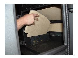
Remove all of the Riddling bars. Lift the side bricks over the side brick retaining strip.
