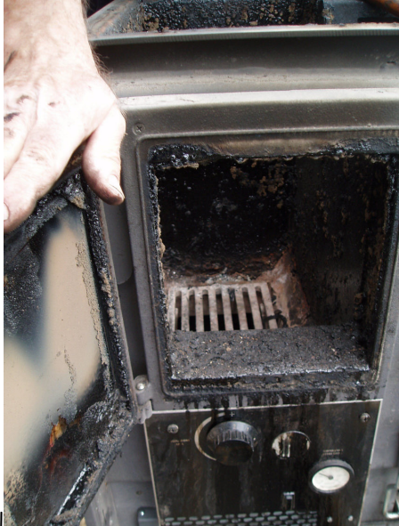
Tar on loading door glass
