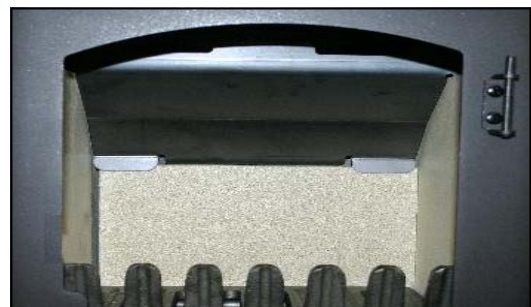
Fig. 3 Liners, throat plate and grate in the Arden
