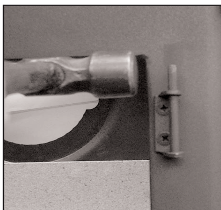
Fig. 9 Adjusting the Camborne hinges
