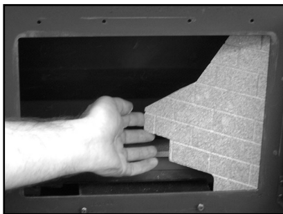
Fig. 3b Fitting the R/H side lining
