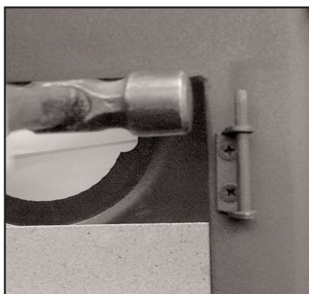
Fig. 9 Adjusting the Arley hinges
