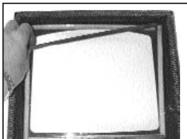
Fig. 6b removing glass retaining bars.
