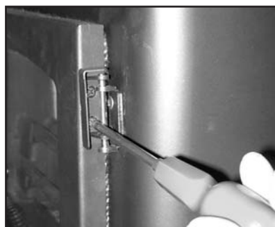
Fig. 5a loosening fire door.
