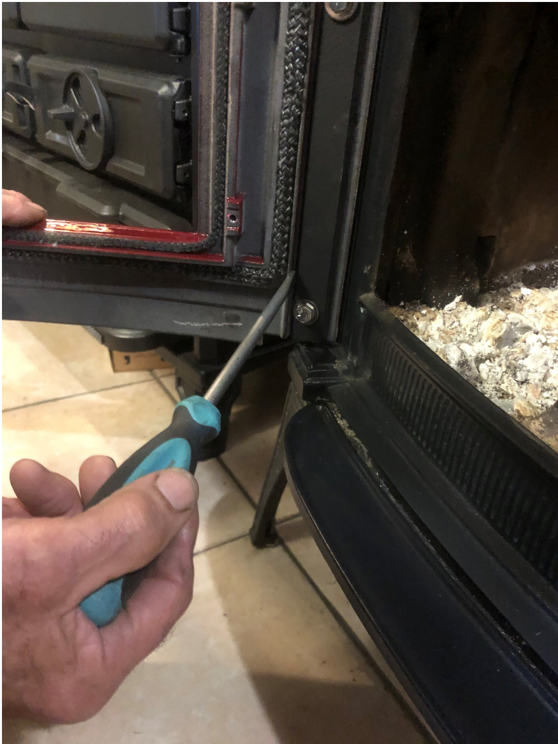
Figure 6 Moves the closed door towards the centre of the stove.
