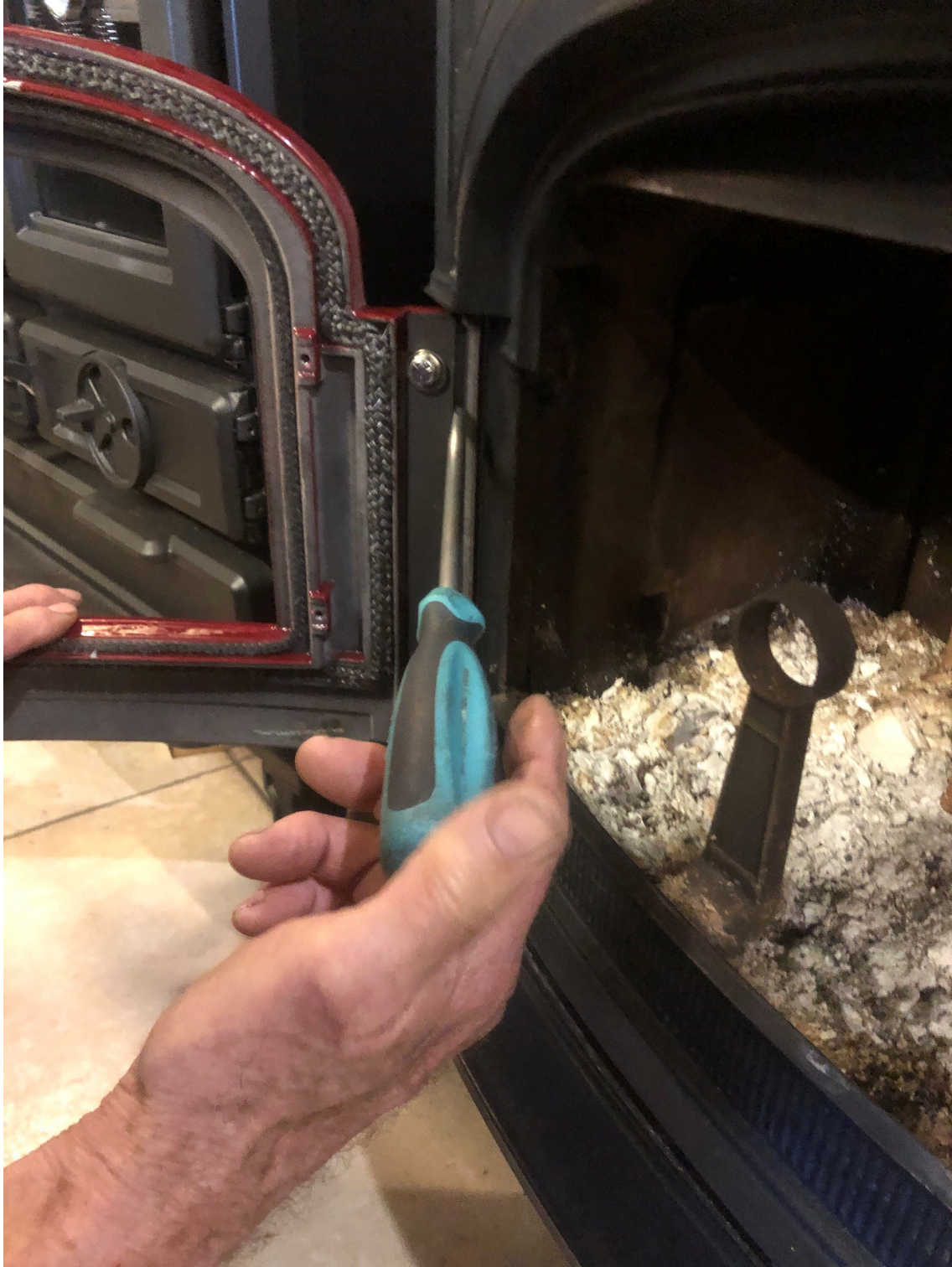
Figure 7 moves the closed door away from the centre of the stove.
