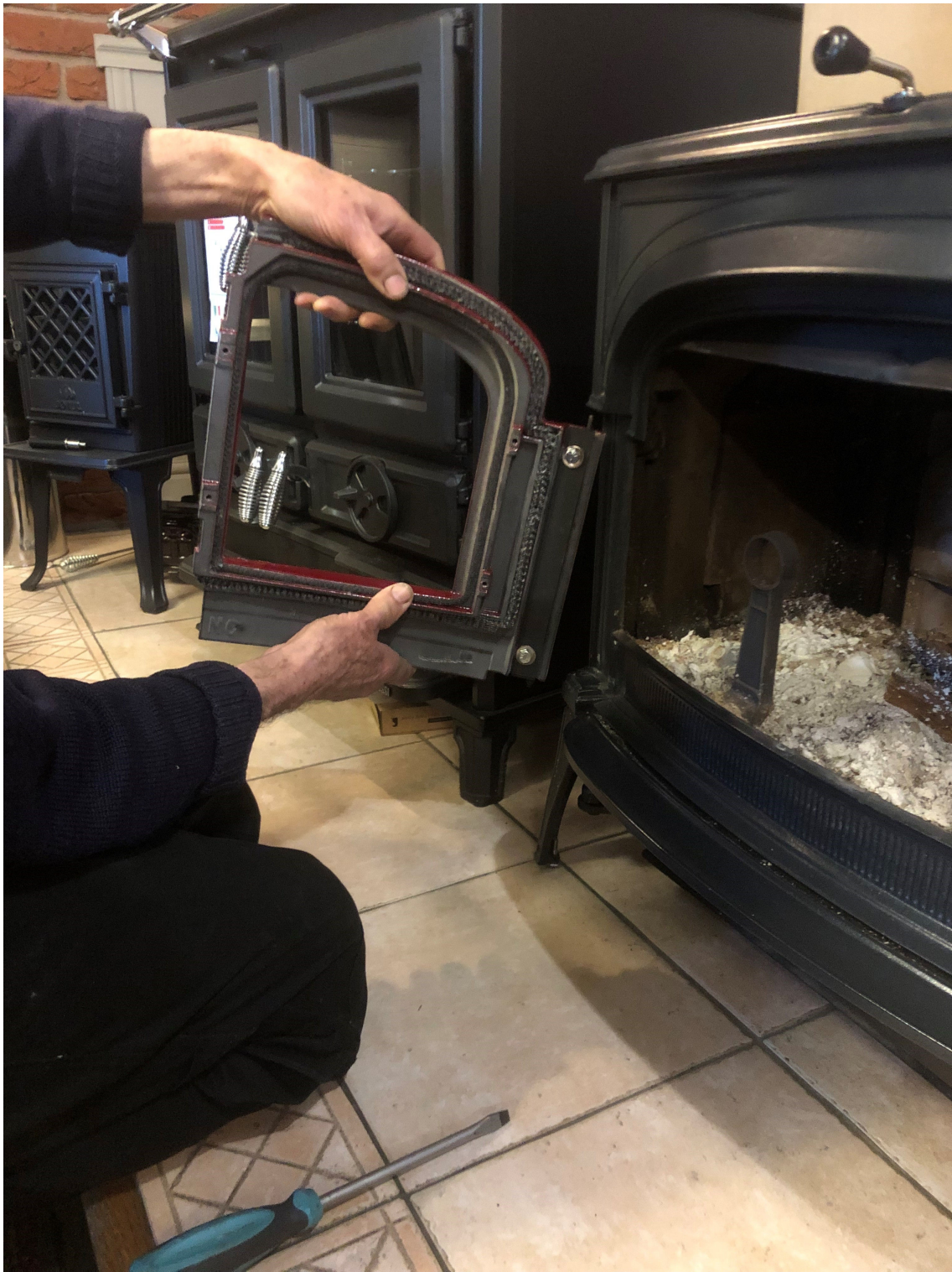
Figure 2 Swing the bottom of the door out and down.
