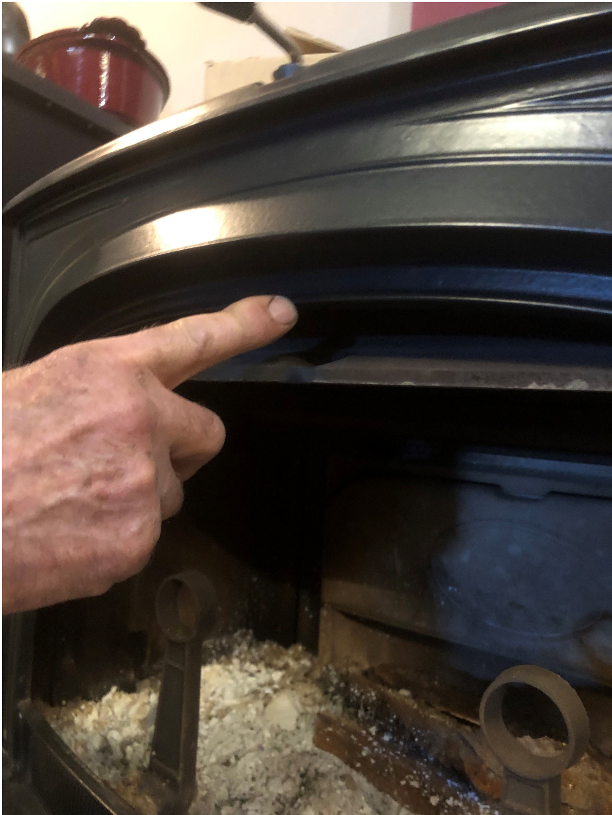
Figure 4 Raised cast edge on to which the rope seals.
