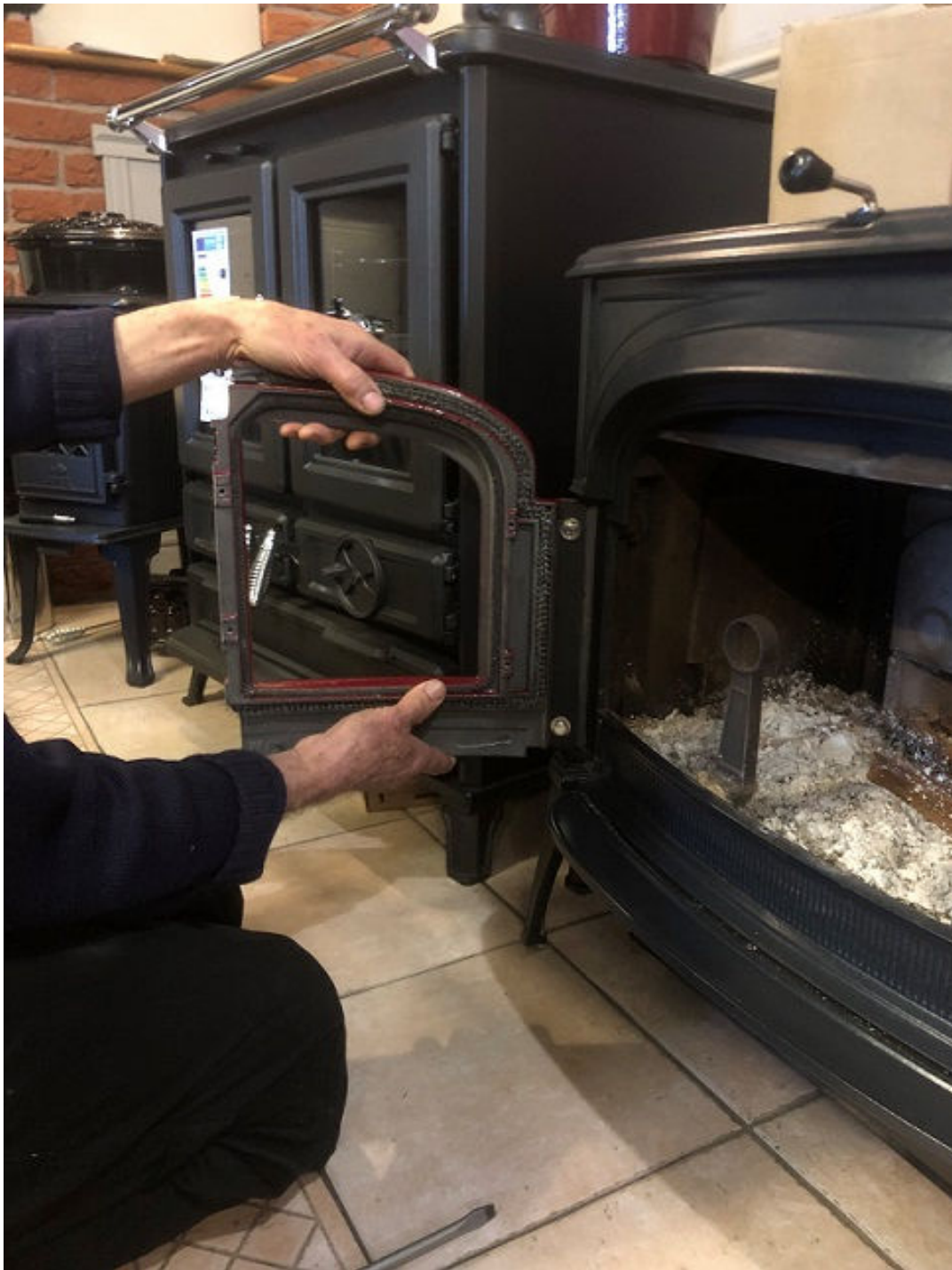
Figure 1 Lift the door off its bottom hinge pin.
