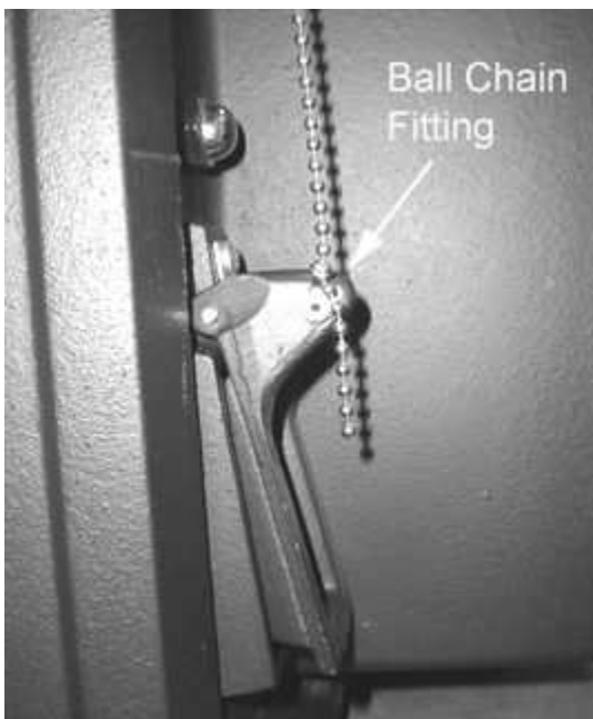
Fig. D-1 Primary Air Valve side view
