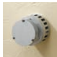
Balanced Flue (No chimney required)
