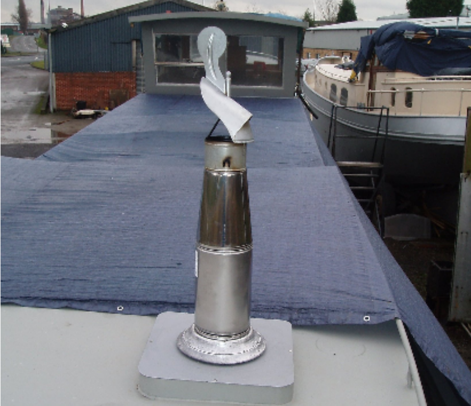
FIG 8 EXTENTION AND TOP STUB 300 EXTENSION AND TOP STUB FITTED
